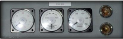
**Step 6.3:** When the synchroscope meter points straight up (12 o'clock position), press the **PUSH TO CLOSE** button on the GEN control panel. **WARNING: Always stand to the side of the circuit breaker when pressing the PUSHTOCLOSE button.**
