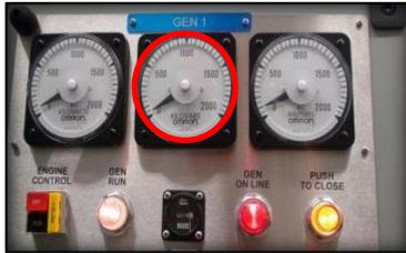
**Step 6.5:** Compare **KVAR** levels of 1<sup>st</sup> GEN & 2<sup>nd</sup> GEN, if not the same, use the **VOLTS ADJUST** knob of 2<sup>nd</sup> GEN to make both KVAR values the same.
